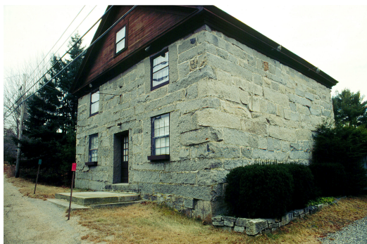
Recent photograph of Stone Store (Source: MDOT)
