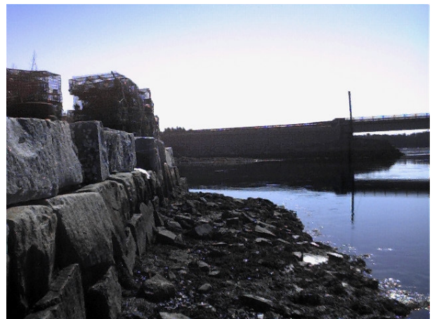
Locally cut granite blocks form pier on Sullivan side of Bay. This pier was once used to load local granite onto ships. Bridge in background (Source: Jim Fisher)
